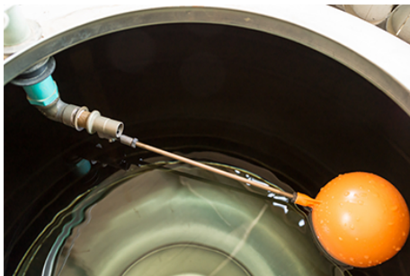
Level control float switch
