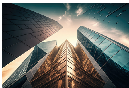
Pressure boosting in tall buildings
